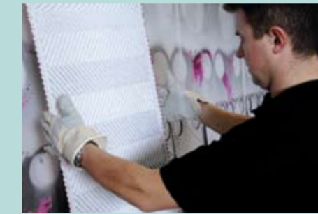
4. Checking the plates for hairline cracks and contact corrosion
